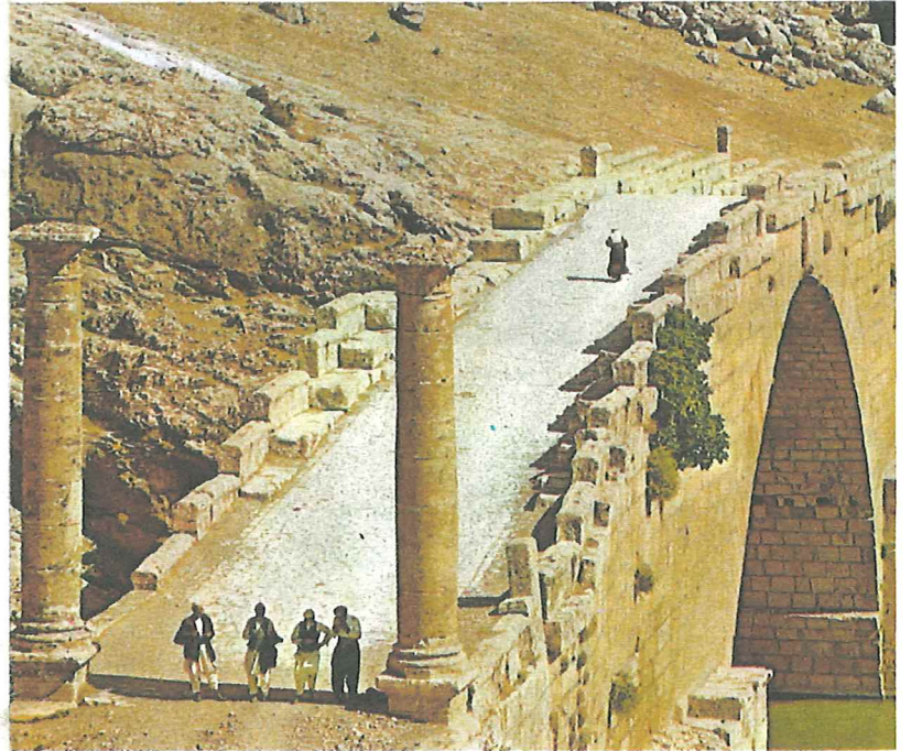
Bridge over the Cendere River near Eski Kâhta
